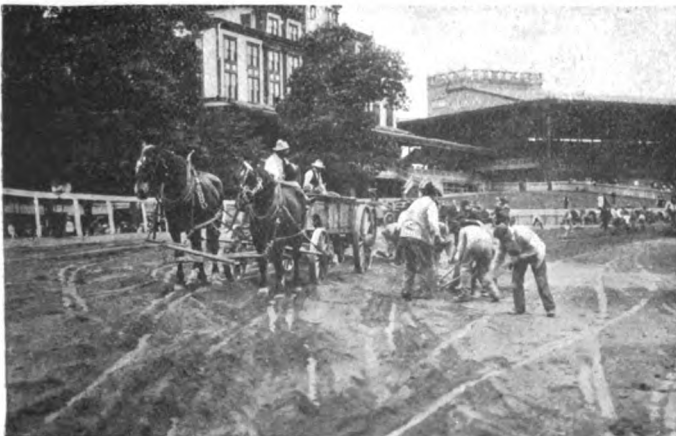
REPAIRING THE MUCH CUT-UP TRACK DURING INTERMISSION.
